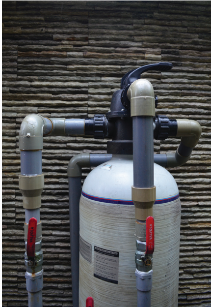
Waterco filters can operate up to 7 bar pressure rating, are hydraulically efficient and can be customised according to customer requirements," Koo explains.
